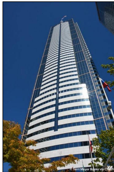
Figura 1-7. Two Union Square Building, Seattle, USA (BOAKE, 200-).
