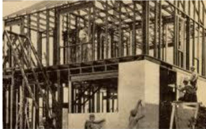
Figure 1.4. Prototype of steel framed residence (DON ALLEN, 2006).
