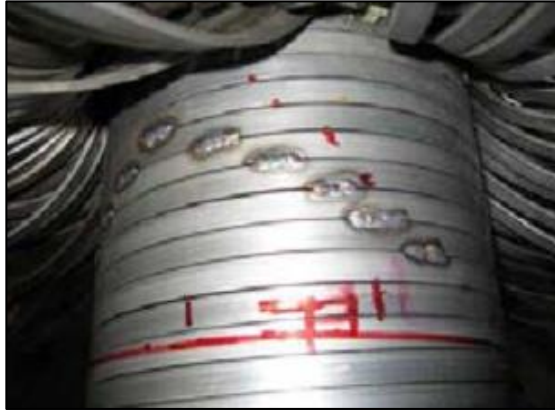
Figure 16. Presusre armour (a) cut and (b) welding. (CAMPELLO, 2014)
