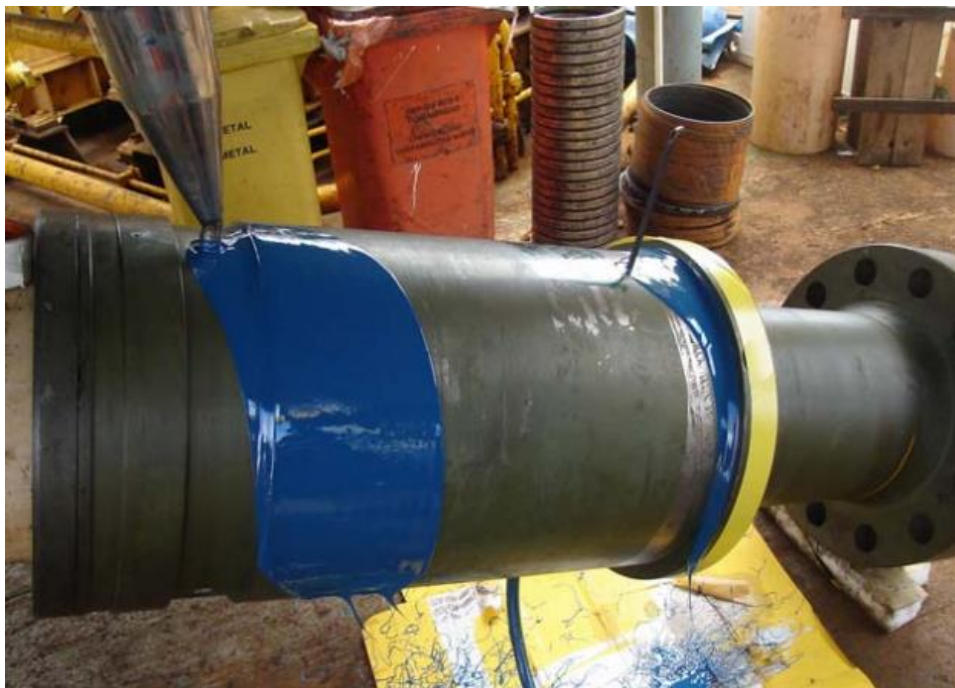
Figure 21. Resin injection after EF mounting (DAFLON, 2010).
