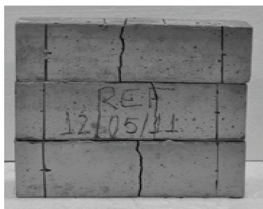
(a) Concreto C0.
